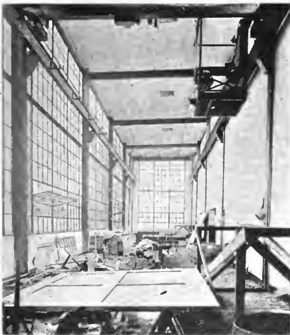
Finishing the floors and ceilings in record time
